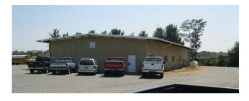
The Bus Transportation building, constructed in 1976, is a metal fabricated building located adjacent to the middle and high schools. The facility is used for bus repair and bus/vehicle parking. There is an adjacent vehicle fueling area, housing below-surface fuel tanks in a containment area and pumps with an overhead canopy.
