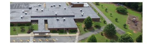
Madison Primary School was built in 1977 and expanded in 1981. The single story is constructed of concrete masonry with brick veneer and is located on 30 acres adjacent to the Hoover Ridge property owned by the County. In the summer of 2010, new concrete sidewalk at the main entry was installed.
